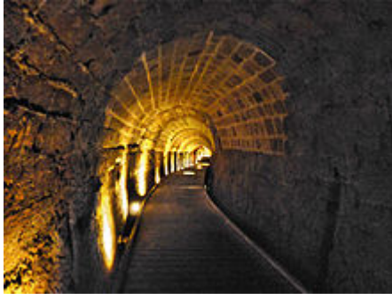
The Templar Tunnel
