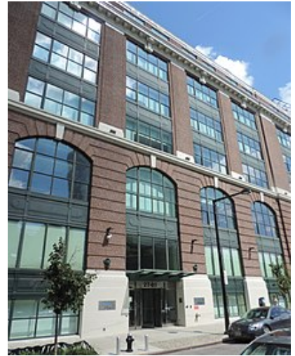
JetBlue headquarters in Queens
