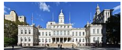
New York City Hall is the oldest City Hall in the United States that still houses its original governmental functions.
