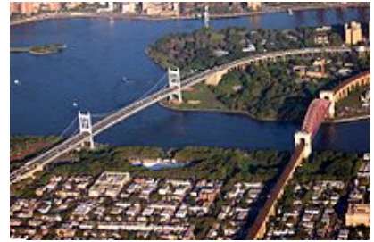
The Triborough Bridge connects Queens with Manhattan and the Bronx.
